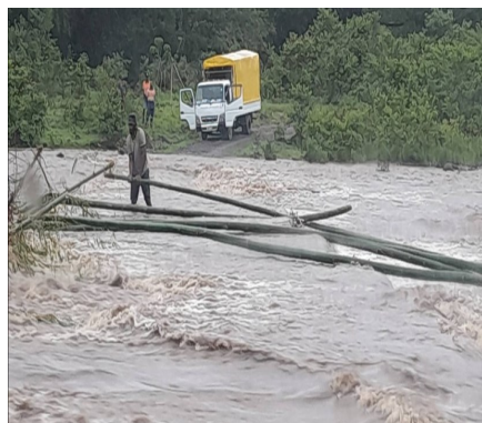
Figure 12b: Matainasau Crossing (Wailao Road) on the 11 th . Source: Fiji Roads Authority.
